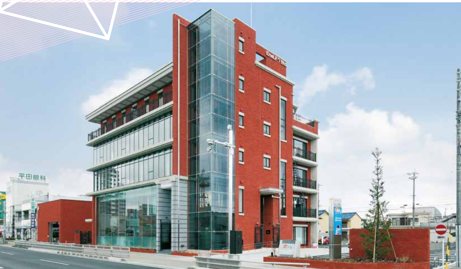
Photo/EneLF7(施工:杉本組)
